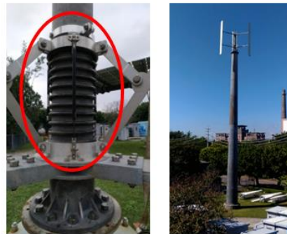
Test of 5 kW VAWT with improved mechanism
